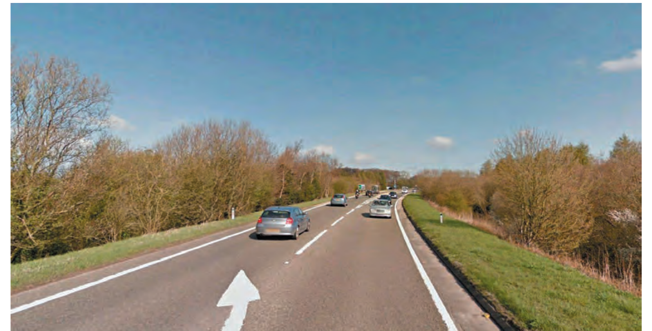
Before: existing A417 between Birdlip and Air Balloon roundabout
